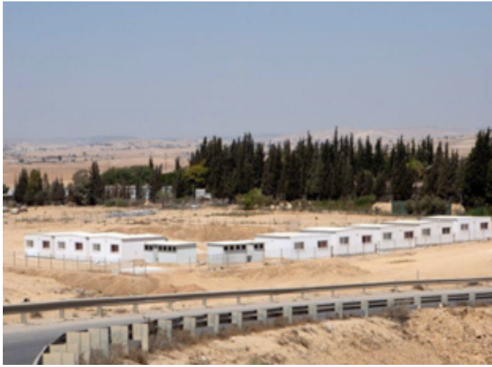
New High-School in Al Zarnug, photography is a courtesy from the village committee
