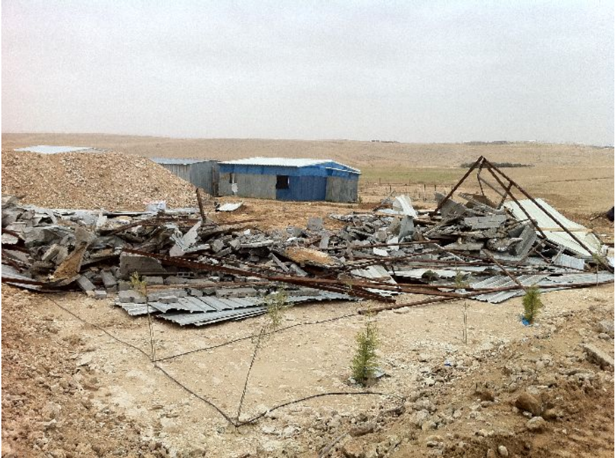
A demolished home in the unrecognized village of Wadi al-Na'am.
