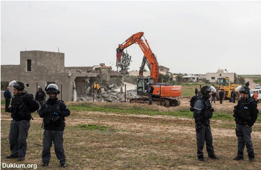
A house demolition near the recognized village of Al-Sayed.
