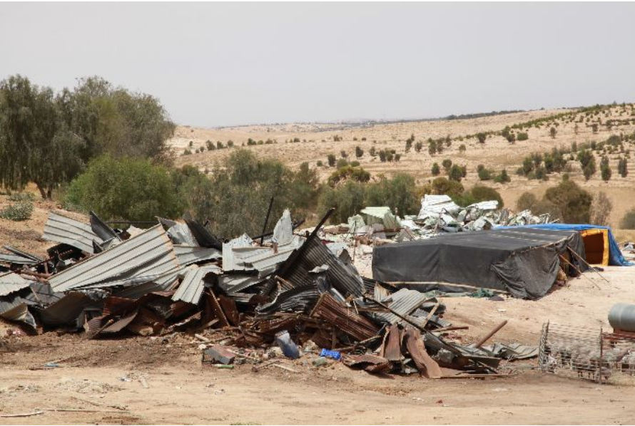
Life continues under demolitions
