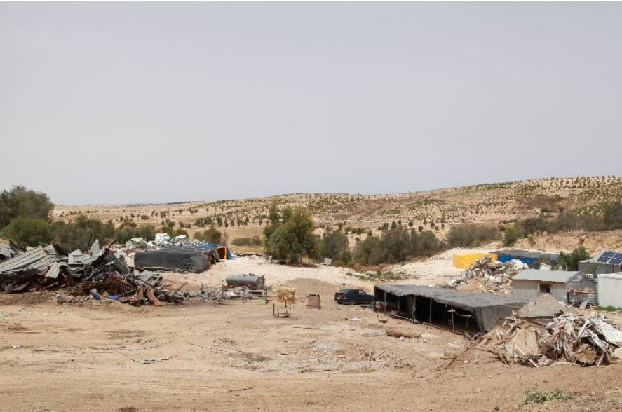
The demolished neighborhood in Atir. The black tents in the picture were built as a temporary replacement for ten houses demolished in this single event.
