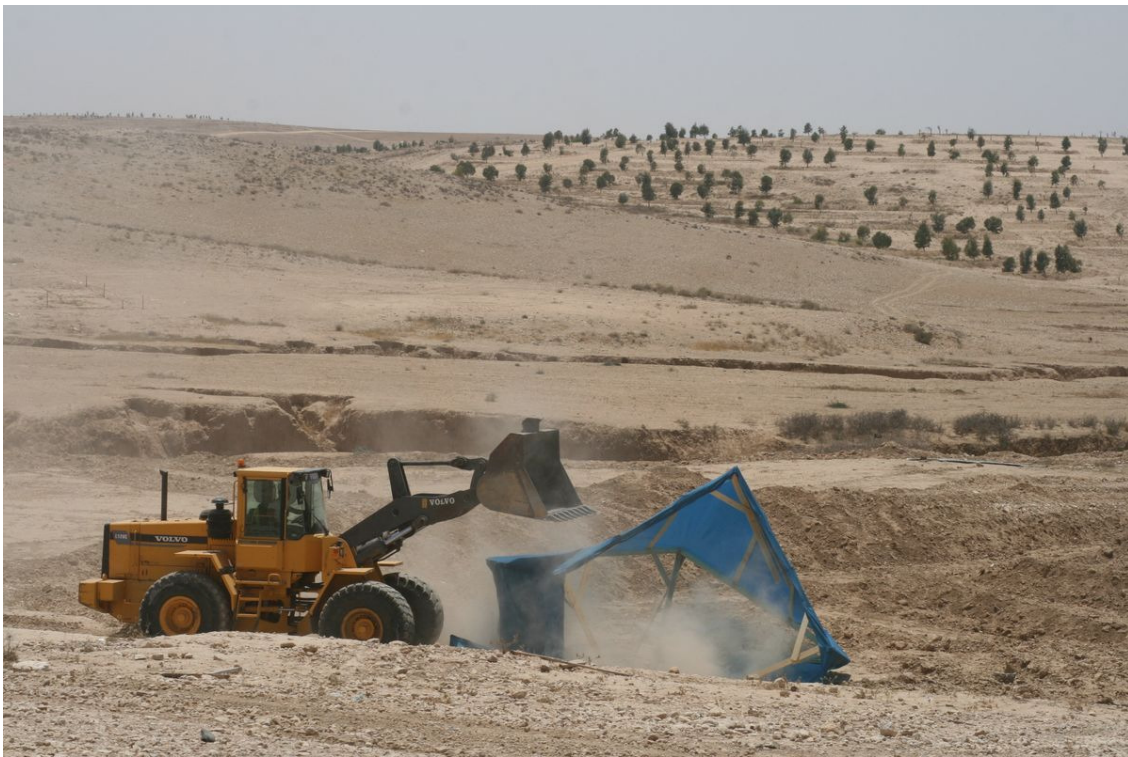
Photograph 2: Demolitions in Al Arakib, 23 August 2011 (photo: NCF)
