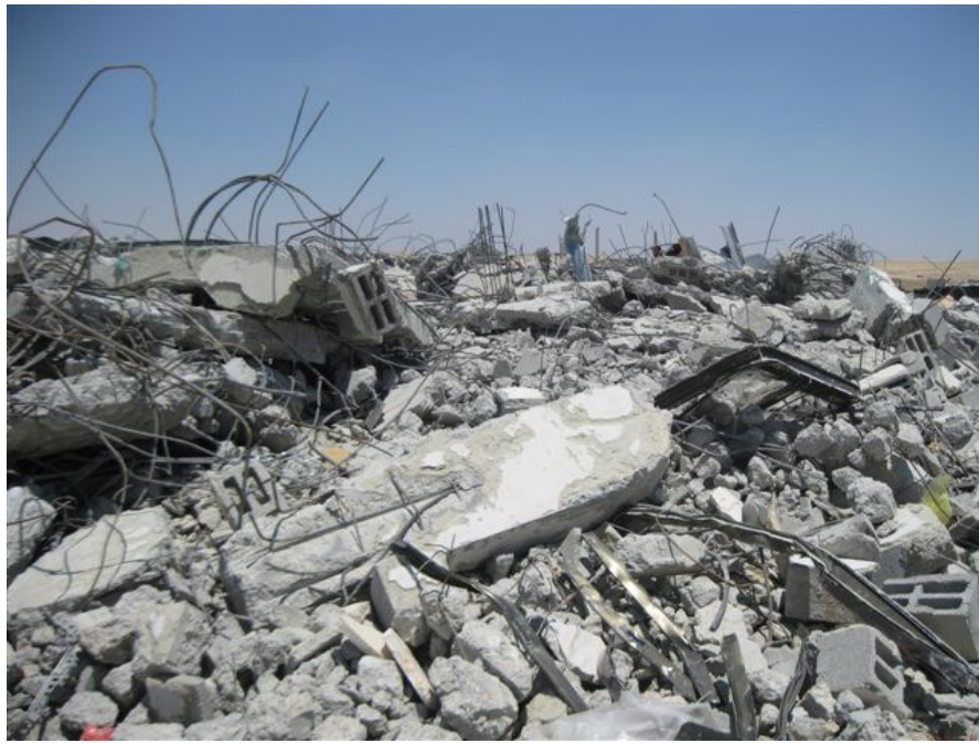
Photograph 1: House demolitions in Al Furah, May 2011 (photo: NCF)
