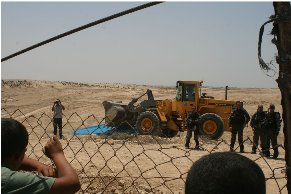
Al Arakib, the 25 th demolition, July 2011 (photo: NCF)
